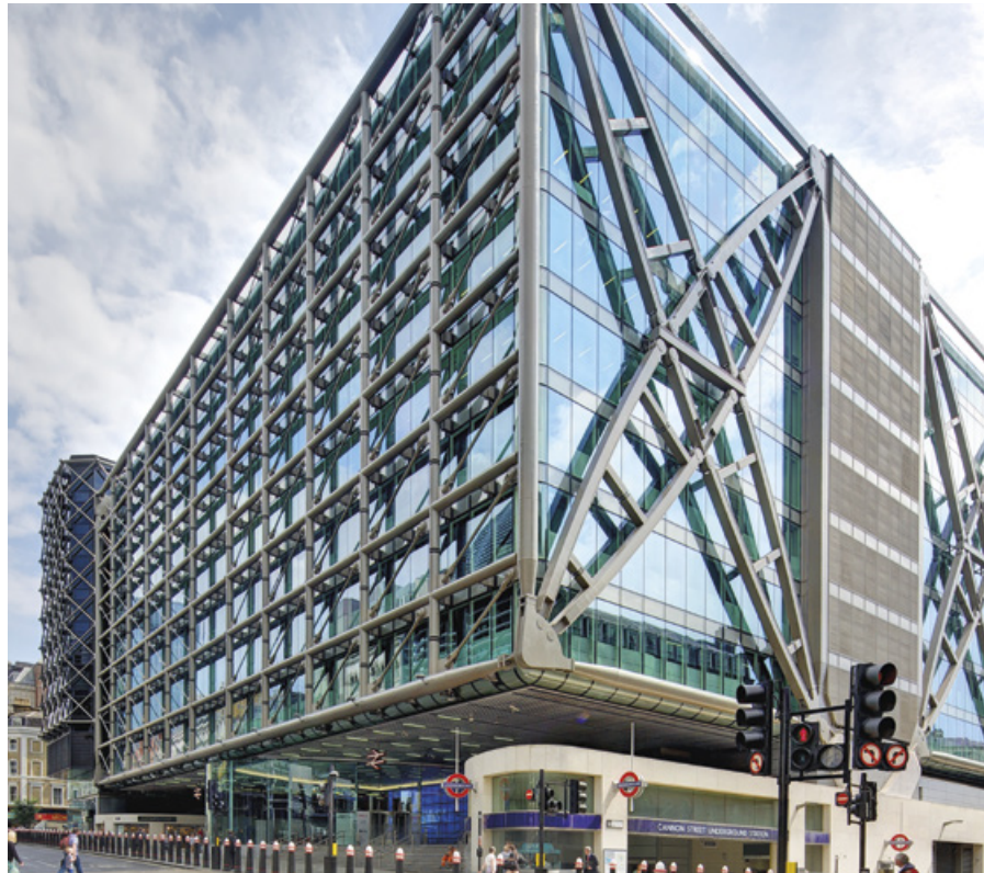
ASDO540-S tie bars M76 to M160 were used as the tension elements in the trusses to form part of this unique and structurally demanding London office building at Cannon Place.
