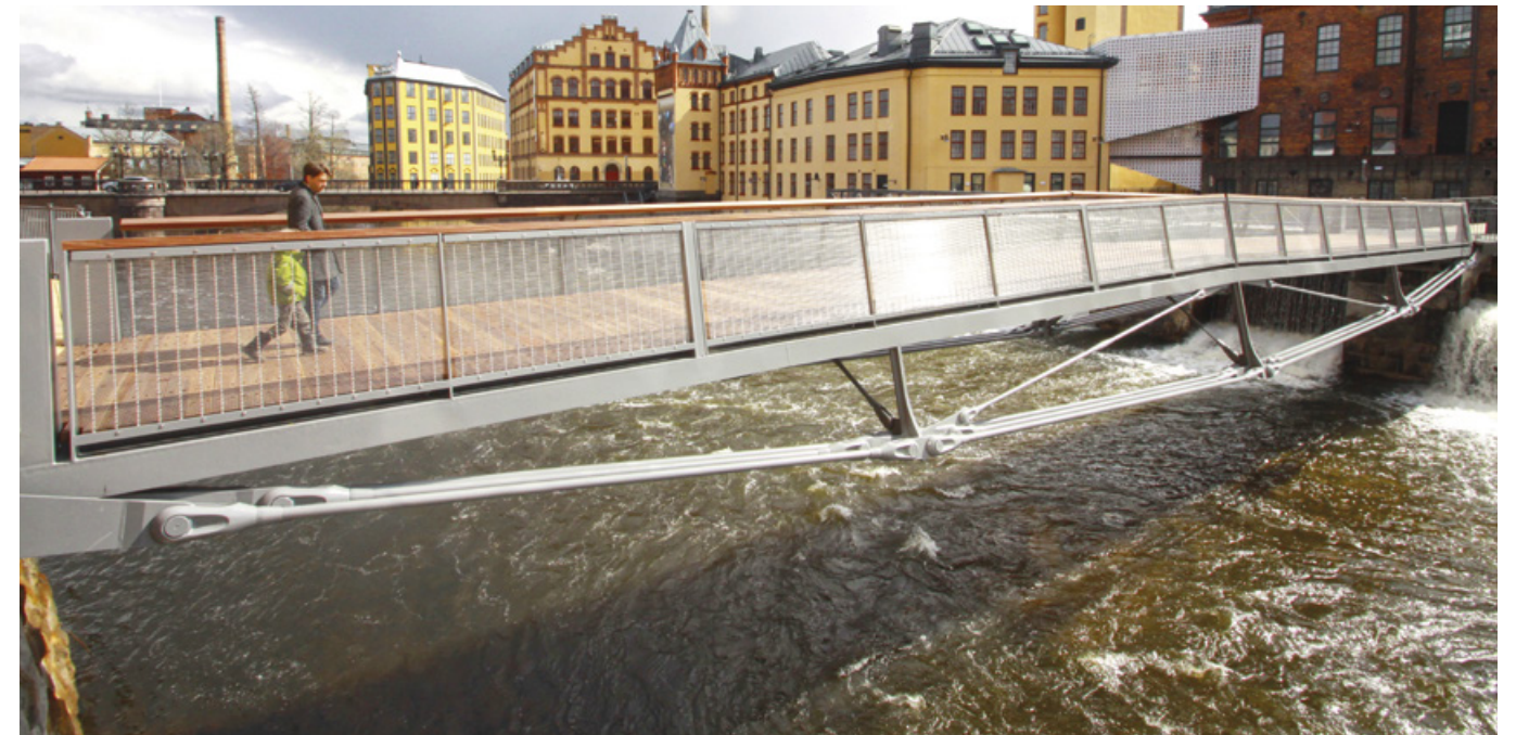
ASDO540-S M56 tie bars were used to form the tension elements for this bowstring truss Kåkenhus footbridge in Norrköping, Sweden.
