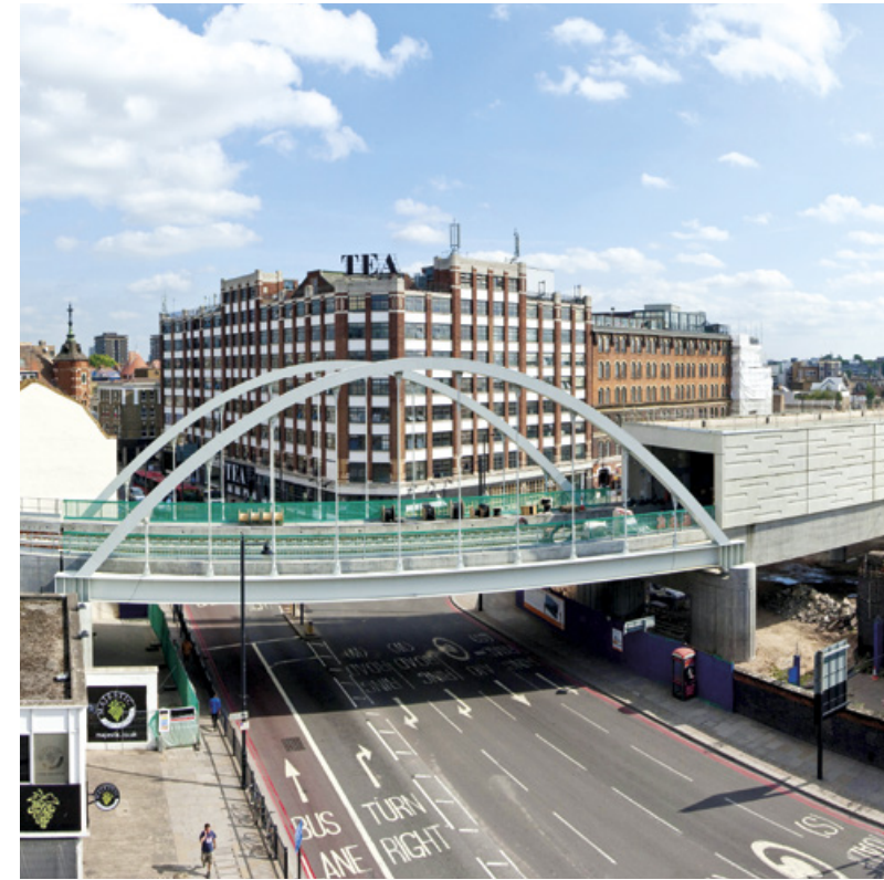
ASDO540-S M90 tie bars are used as hangers on this East London Line railway bridge in Shoreditch. As well as undergoing rigorous QA the system was also fatigue tested to 2m cycles.
