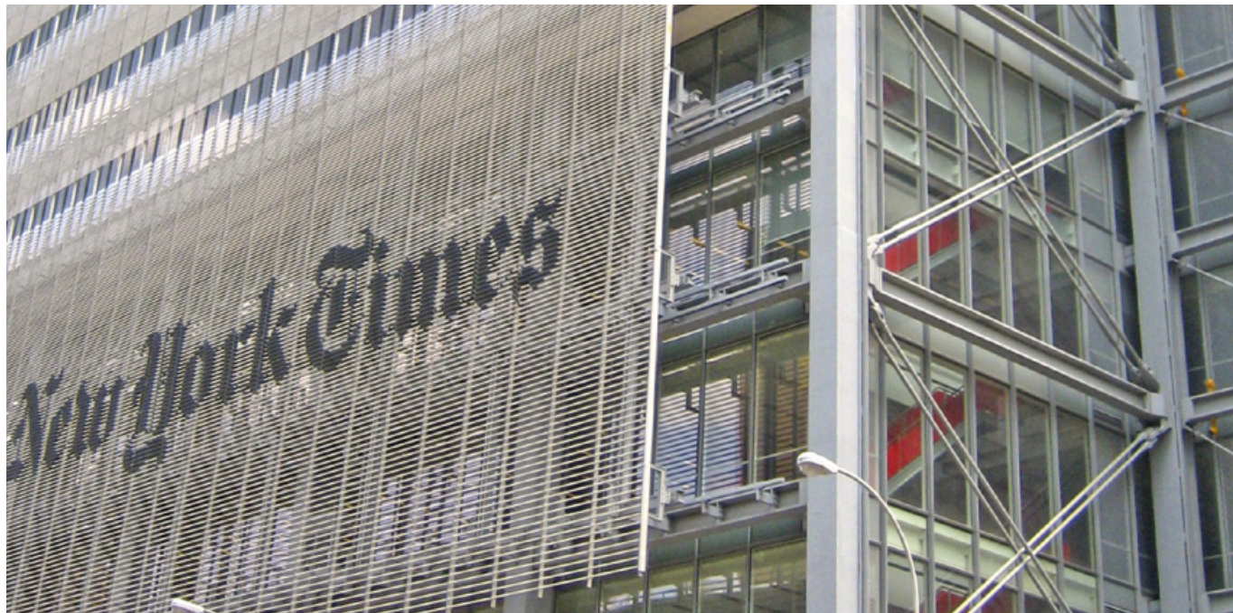
Tandem ASDO540-S bars were used to brace the new 52 floor headquarters for the New York Times newspaper.
